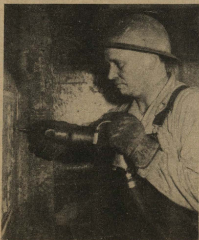
BOBS SEAM Mike Vivier, tank test day shift, bobs a weld seam in tank adjacent to that being tested. Welders will follow him to close leaks securely. (Swan Island photo)
