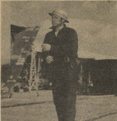
Travel Rotating his hands and arms, Leadman Rigger D. S. Attebery of Vancouver signals the crane operator to keep moving, a part of riggers' sign language.
