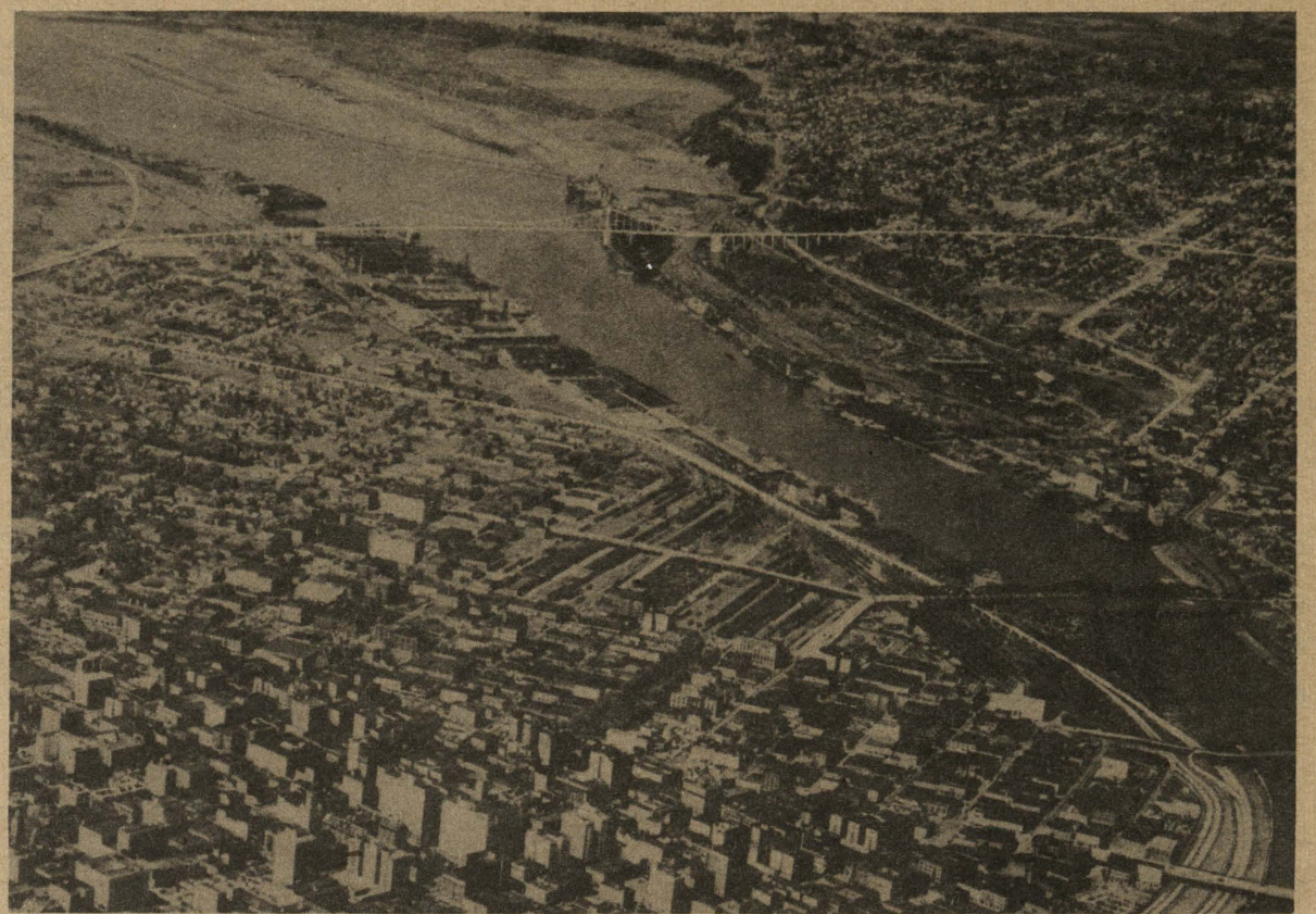
Thruways Biggest chunk of the Moses Plan is a proposal for arterial thruways along Portland's west side connected with a similar east side thruway by a new bridge east of Swan Island. This engineer's drawing on a prewar aerial photo also shows a proposed elevated thruway connecting with present harbor drive.
