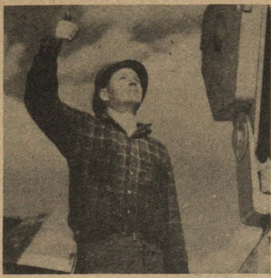
Boom Up Rigger Marvin Bragee, Vancouver, isn't trying to hitch a ride to heaven. He's signalling the crane operator to raise the boom.
