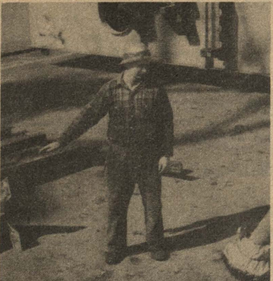
Stop Like an umpire calling a man safe on first, Vancouver Rigger Marvin Bragee tells the operator to stop. Both arms would mean an emergency stop!
