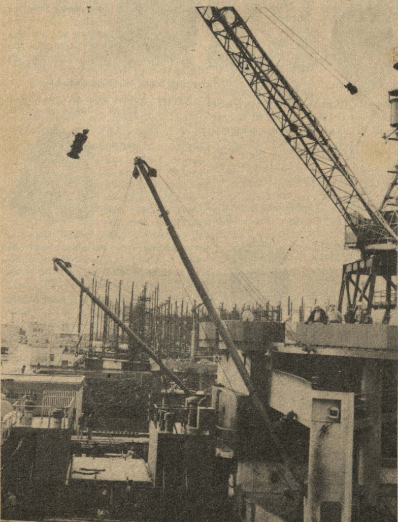
Disarmament Those smoothly working guns aboard the Vancouver-built C-4, SS Marine Falcon, are removed at Swan Island to be crated and stored by the navy. In picture a gun director is swung to the shore by a whirley crane. (Swan Island photo)
