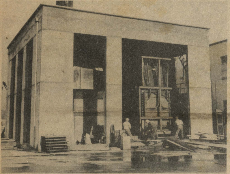
Steam From Surplus When the tanker contract cutback came following V-J Day, boilers for Hull 154 were declared surplus. One of the twins was brought into use when it was installed as the second boiler in the shore steam plant for the Swan Island Repair dock operations to furnish live steam to vessels at the dock. Riggers installing boiler are, (from left), C. B. Burt, Ben Laughlin and Don Painter. (Swan Island photo)
