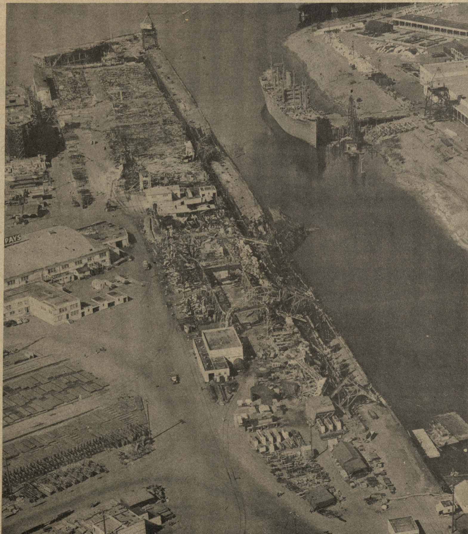
Fire Ruins Viewed This aerial view of Oregon Ship's Outfitting basin and adjoining buildings shows the complete devastation wrought by the recent fire. The Mold Loft, which had a close call from the blaze, can be seen at left. Across from the ruins, new outfitting facilities are pictured with a Victory cargo ship tied up to the dock. Additional ships are moored at the yard's dolphins, shown just north of the inlet to the Outfitting dock.
