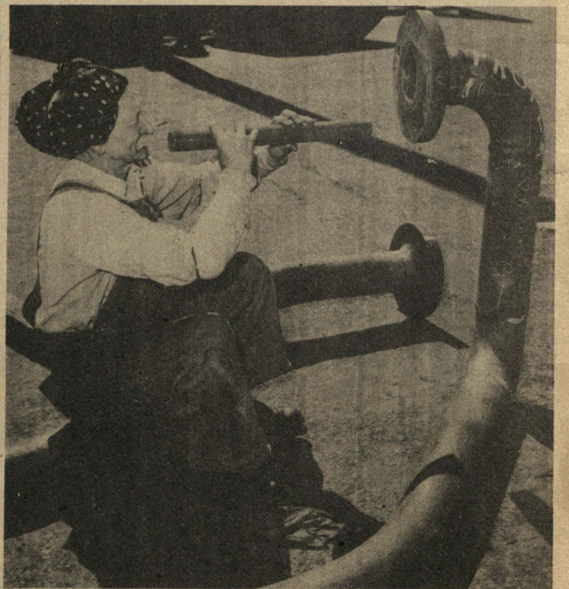
Corny Cobra Henry E. Holum, pipe tester, practices a little hokus-pokus on a main steam pipe that looks like a giant snake. Holum says this isn't the way he tests pipes. (Swan Island photo)
